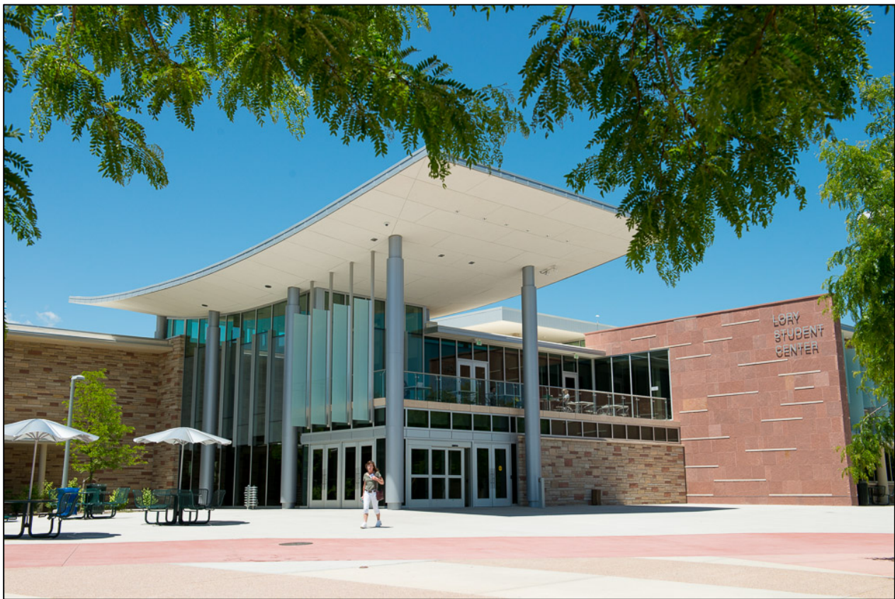
The revitalized Lory Student Center features numerous energy efficiency upgrades, including: smart glass, energy-efficient lighting and lighting control packages, low-emissive glass, overhauled mechanical heating and cooling systems, low-flow fixtures and water-efficient appliances, and high-performance insulation on all perimeter walls.
